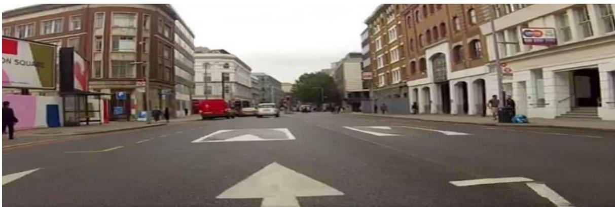
*Figure 4: Optical illusion speed bumps on a London road (BBC, 2016).*
